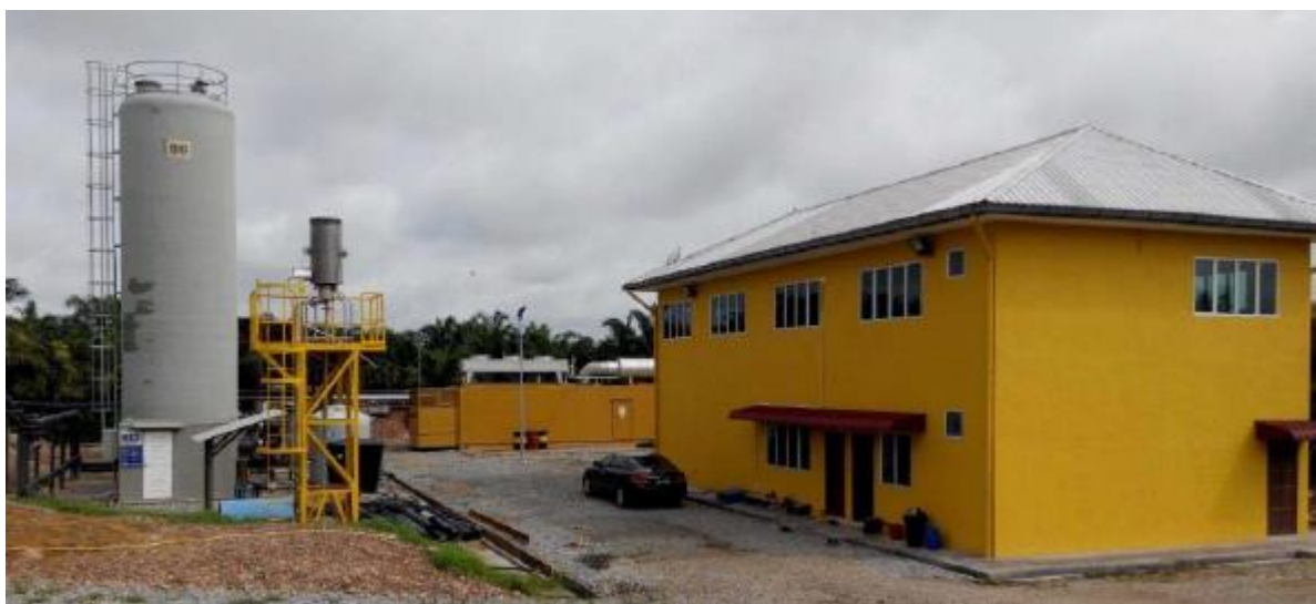
Figure 26: Jeng Huat Kemayan project: Site overview.
