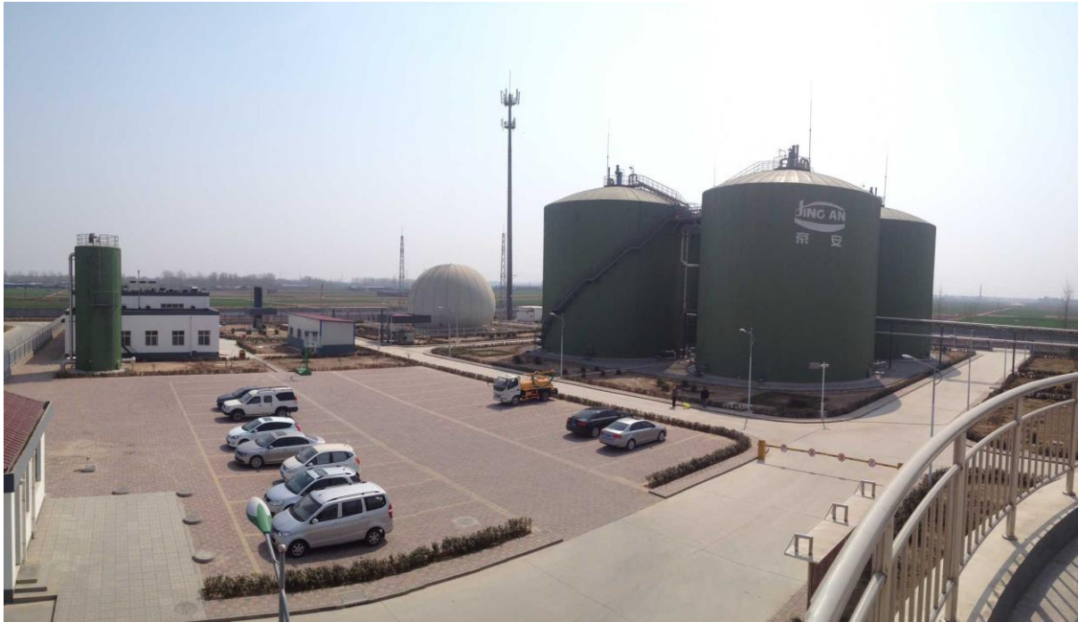
Figure 9: YFJA HeBei Province project: Overall view of site.
