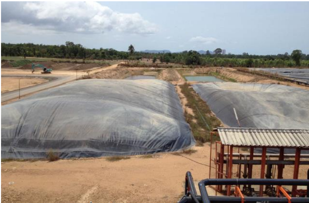
Figure 27: TQS Kanchanaburi project: Lagoon digesters.
